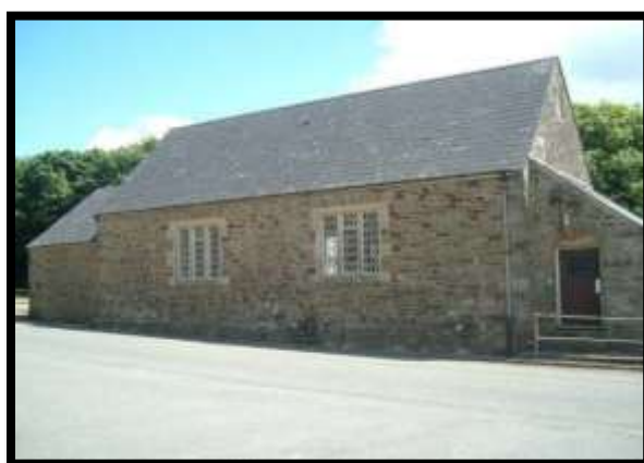
The old Victorian village school, vacated in September 2004 for our new building.
